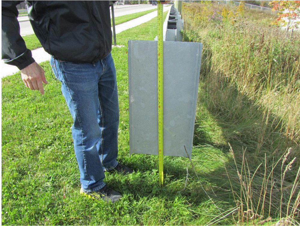
Figure 60: View showing the installed height of the end plate with the base positioned 10.5 inches above the ground.
