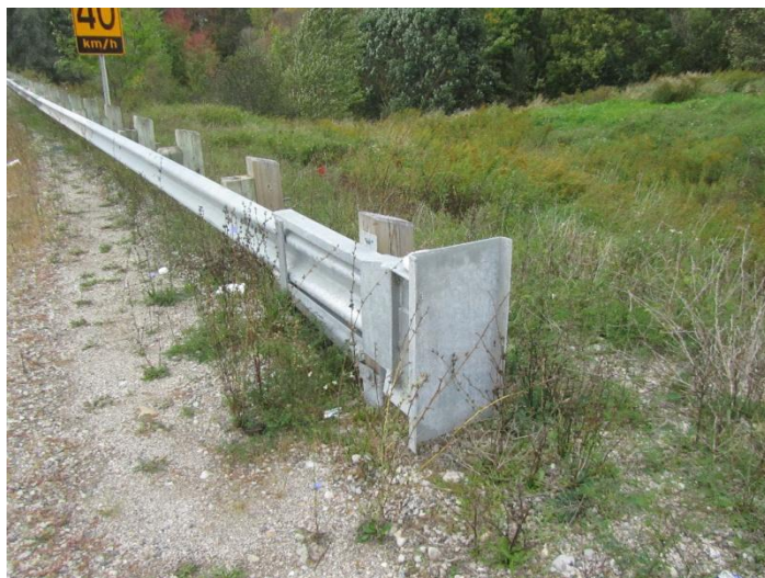
Figure 1: View of end cap of west guardrail. Evidence suggests that the original end cap was damaged and replaced by the current one which has a 4 inch wide channel.
