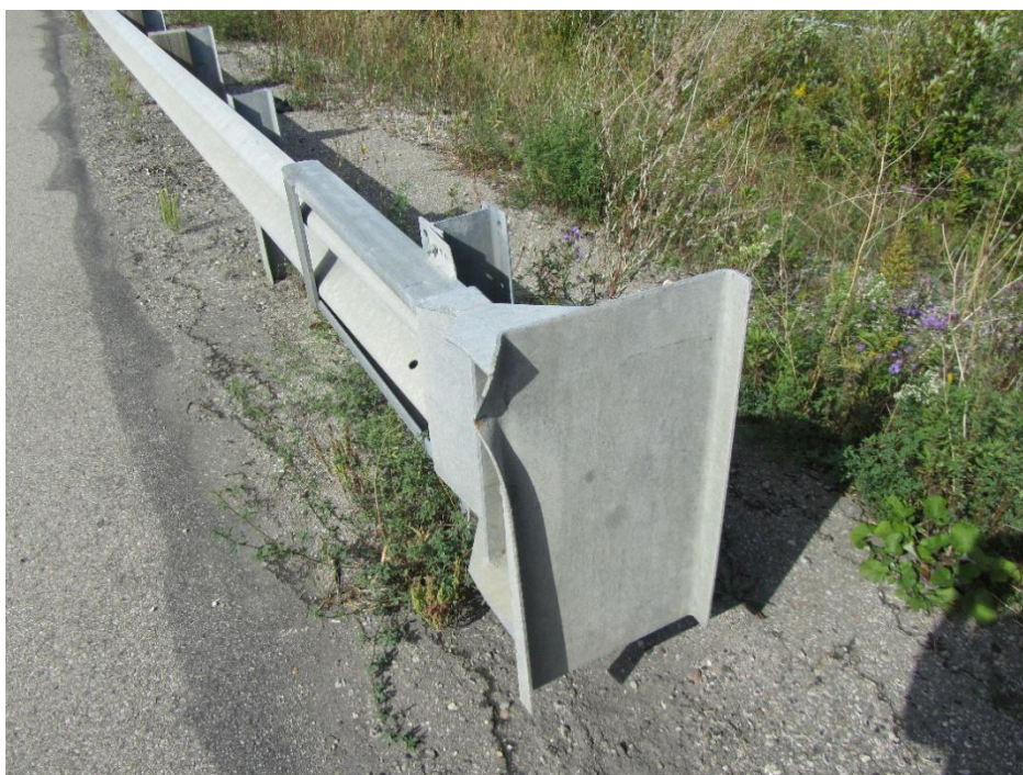
Figure 41: View of damage evidence to face of end plate.
