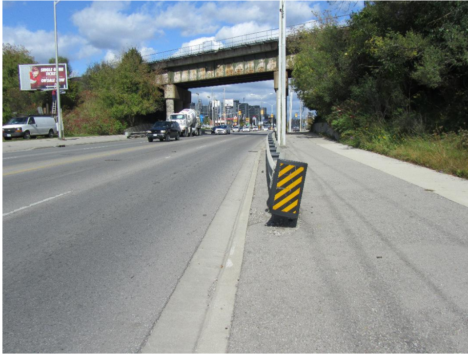
Figure 115: Overall view of 2nd End Cap of east guardrail. Note that the end plate is on an obvious non-vertical angle.
