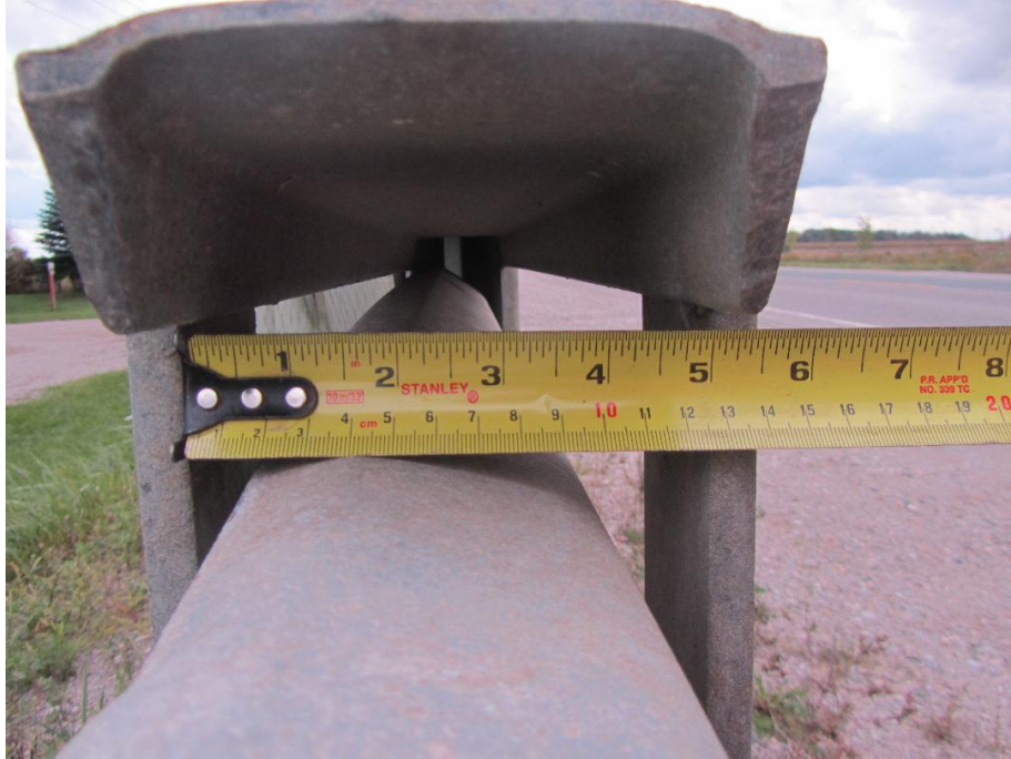
Figure 27: Measurement indicates the channel is 5 inches wide.
