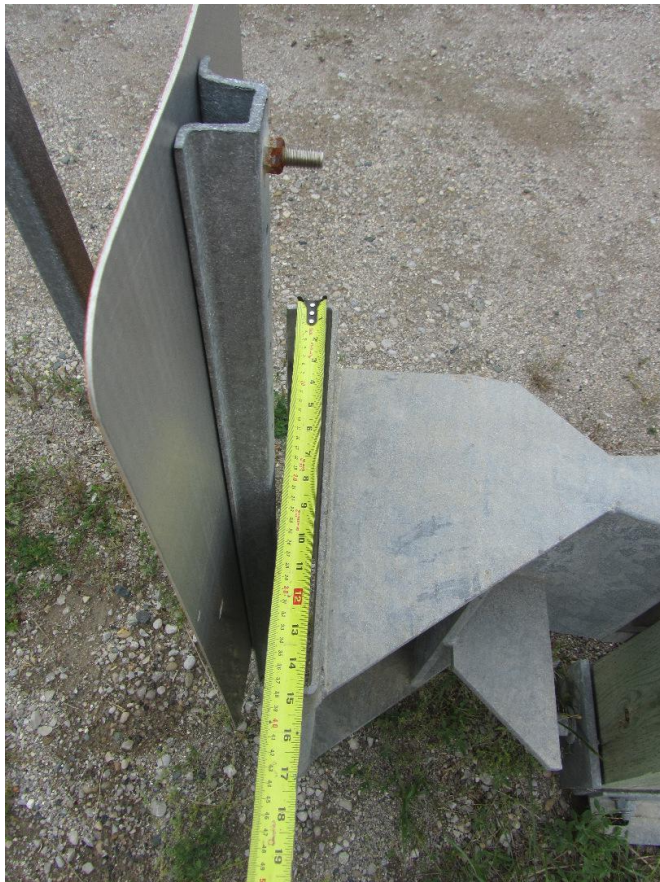
Figure 28: Without the black cover the end plate is about 15 inches wide.
