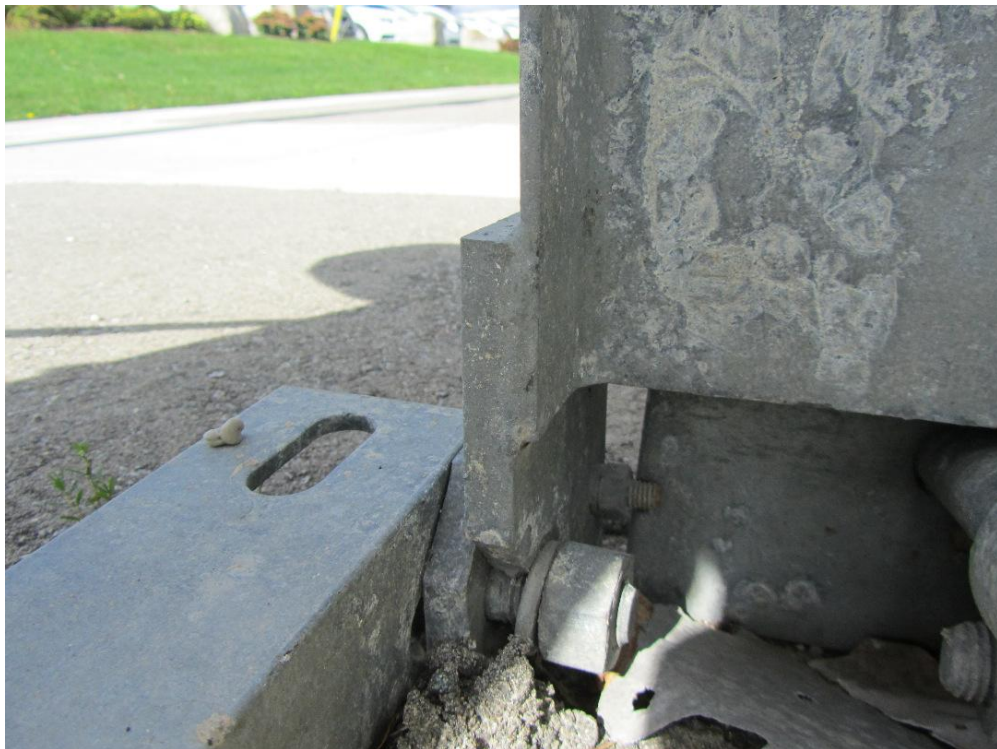
Figure 144: View showing the press fit of the base of the vertical anchor post just behind the end plate.
