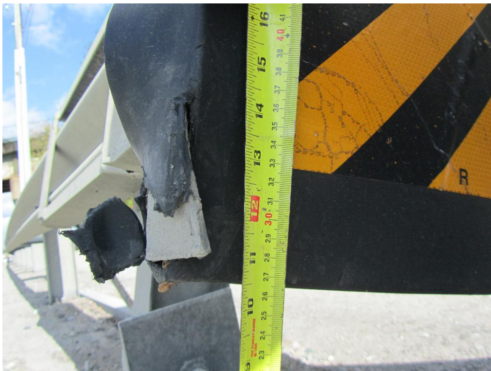
Figure 122: View indicating that there is impact damage to the bottom, street side corner of the end plate.
