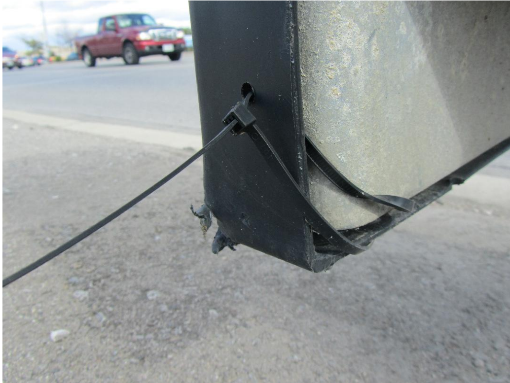
Figure 137: View of typical plastic tie used to hold the plate cover onto the end plate.
