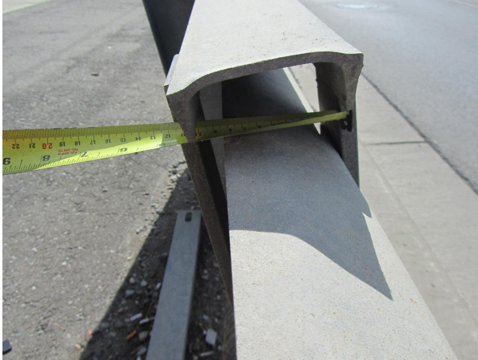
Figure 125: Measurement indicating that the channel is 4 inches wide. Note that the rail within the channel is resting at a low position.
