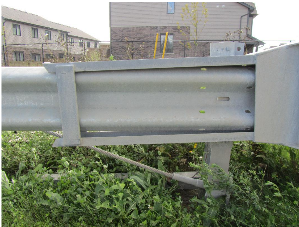
Figure 49: Closer view of channel and guardrail beam noting that they are not in vertical alignment.
