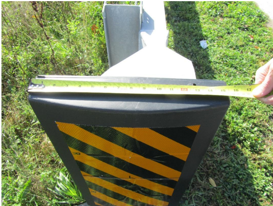
Figure 71: Measurement indicating typical width of 15.5 inches to the cover the end plate.
