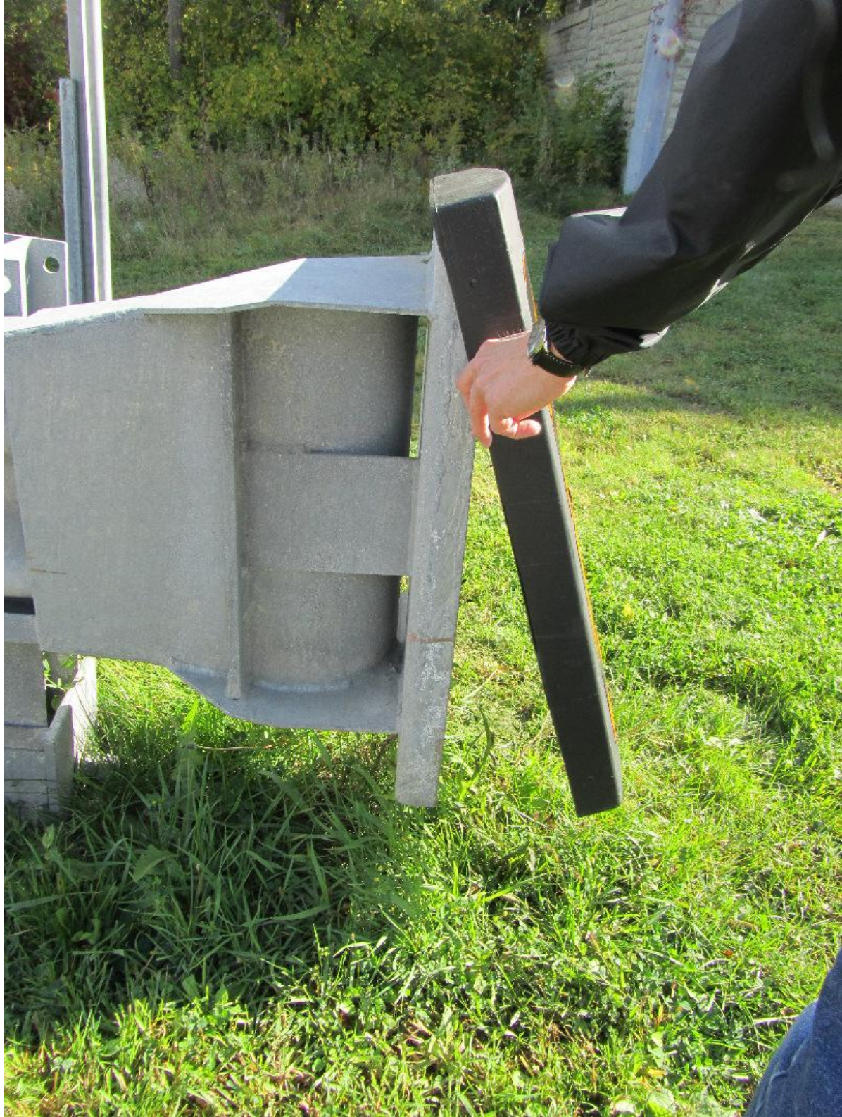
Figure 90: Because there are no plastic clasps to secure the cover to the end plate the cover can easily become dislodged from its position.
