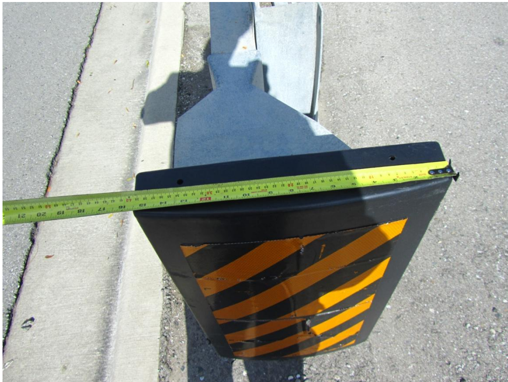
Figure 104: measurement of end plate cover indicating the typical width of 15.5 inches.
