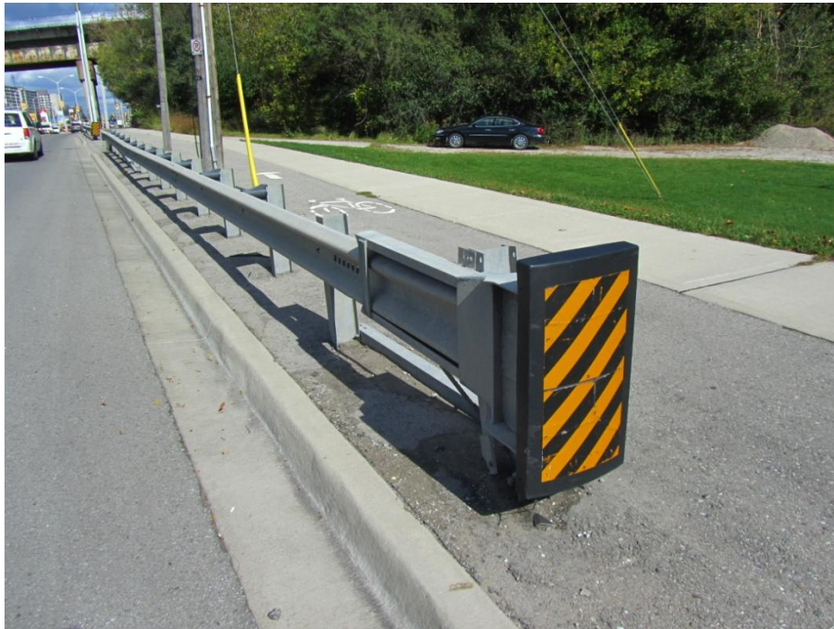
Figure 101: Overall view of 1st south end cap of the east guardrail. The 2nd south end cap is visible in the distant background.
