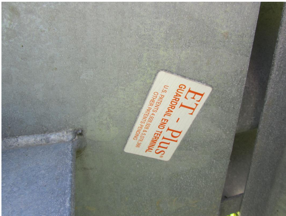
Figure 96: View of tag attached to the end plate indicating that this is one of the ET-Plus terminals that is the subject of the defect allegations.
