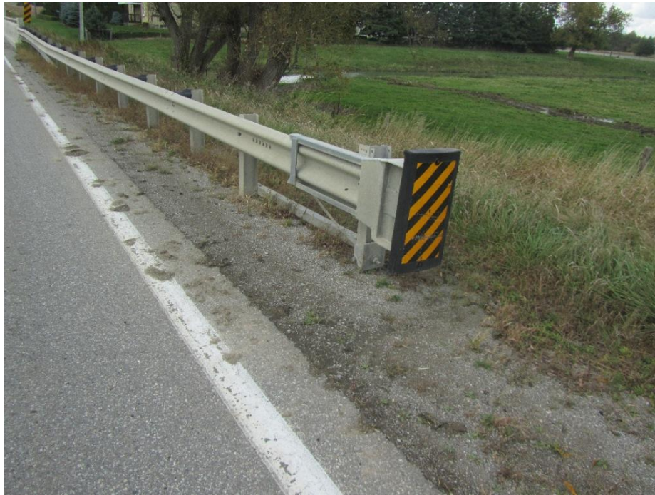
Figure 15: Overall view of end cap of north guardrail.
