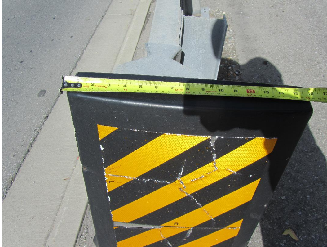
Figure 119: View showing that the end plate cover is the typical width of 15 inches.
