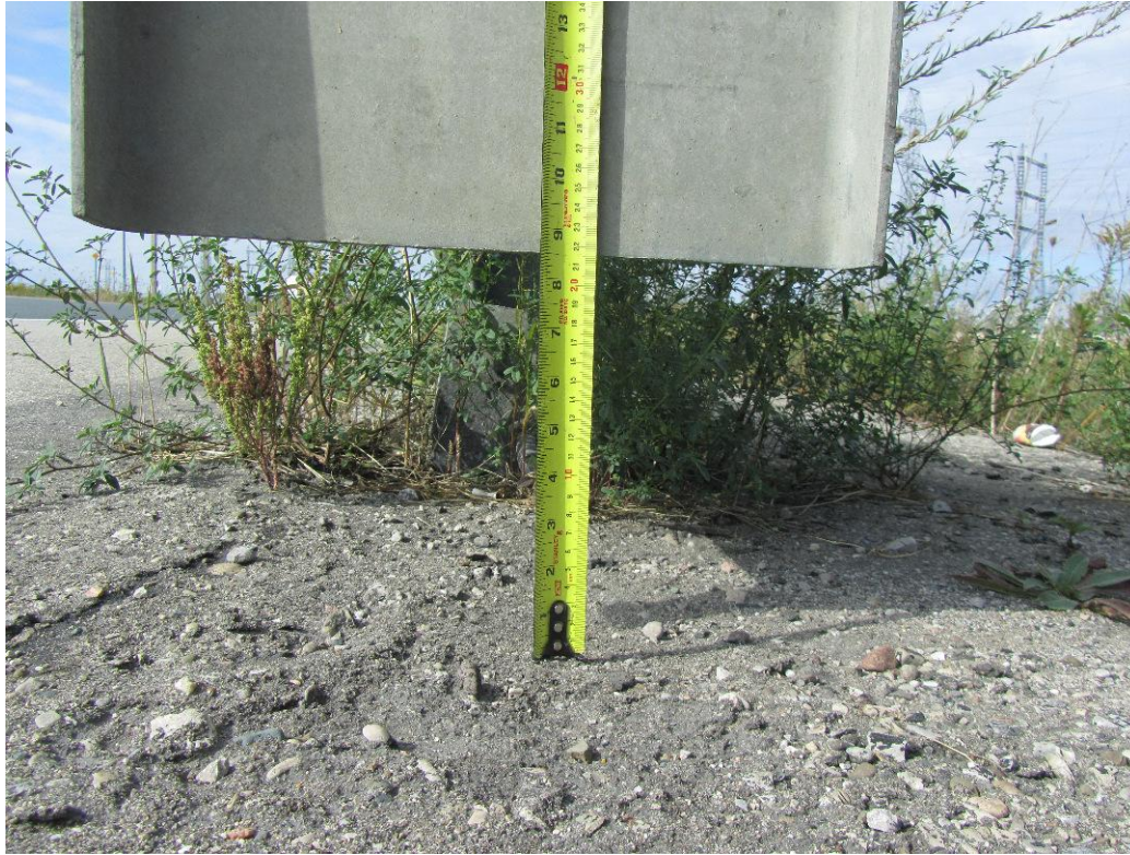
Figure 42: Base of end plate positioned about 8.5 inches above the ground.
