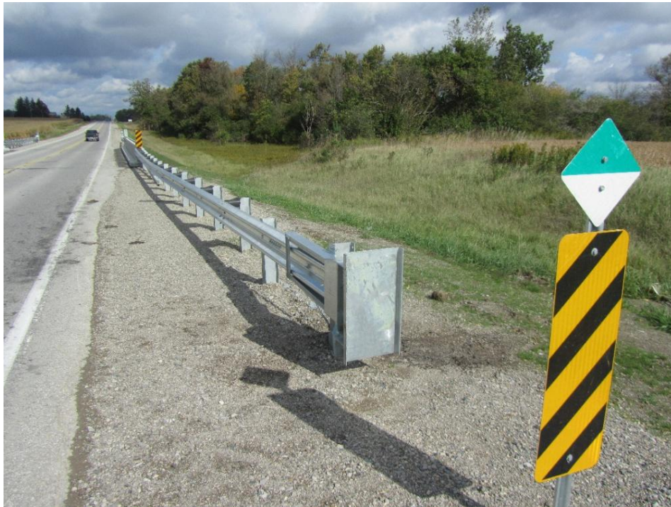
Figure 11: Overall view of east guardrail with end cap that is missing its front cover.
