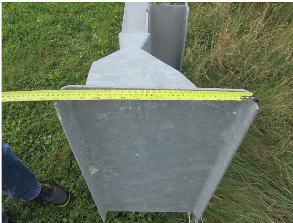
Figure 59: Measurement indicating the typical width of 15 inches for the end plate.
