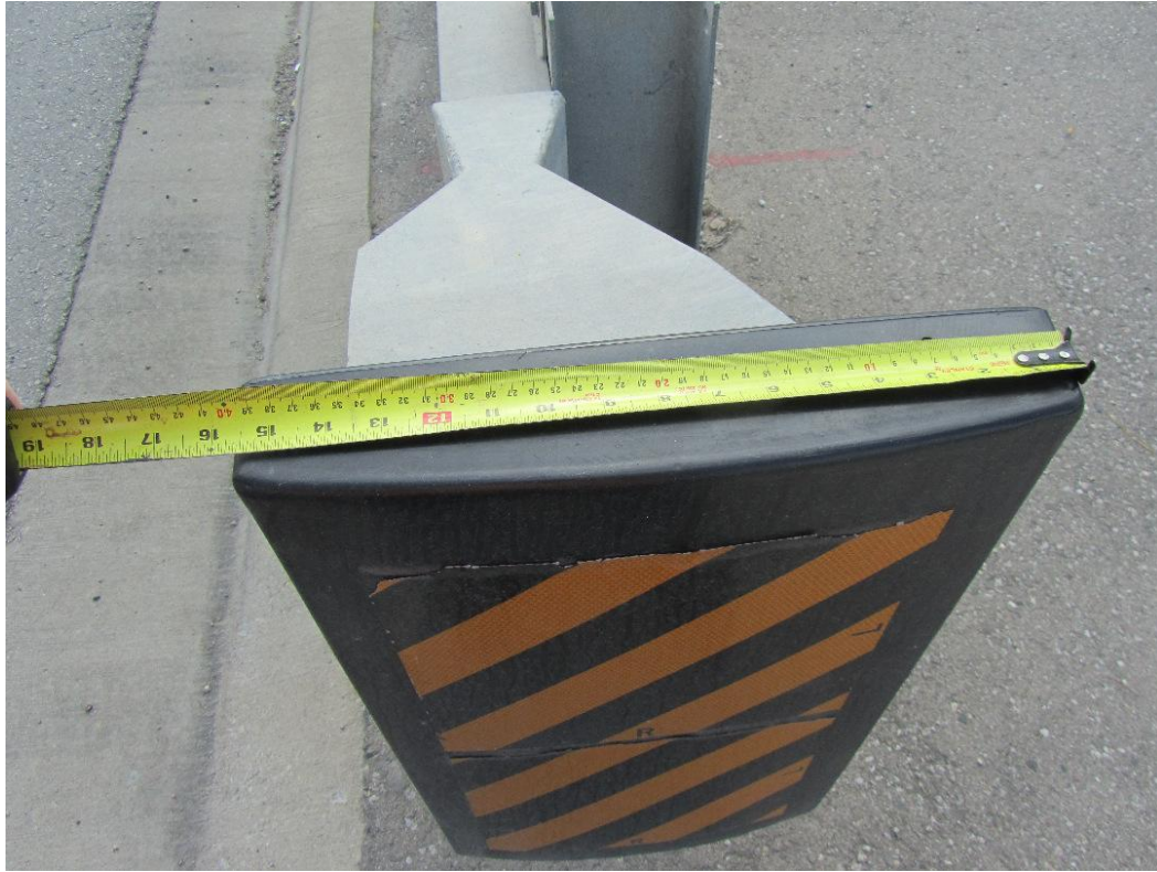
Figure 141: Measurement indicating that the end plate cover is 15.5 inches wide.
