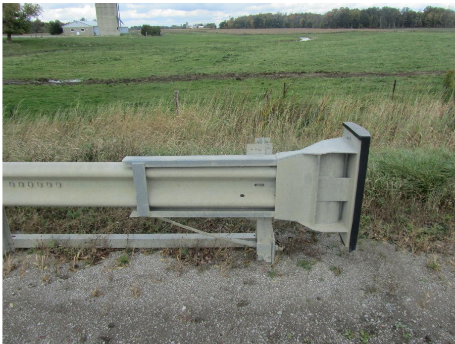
Figure 16: Street side view of end cap.
