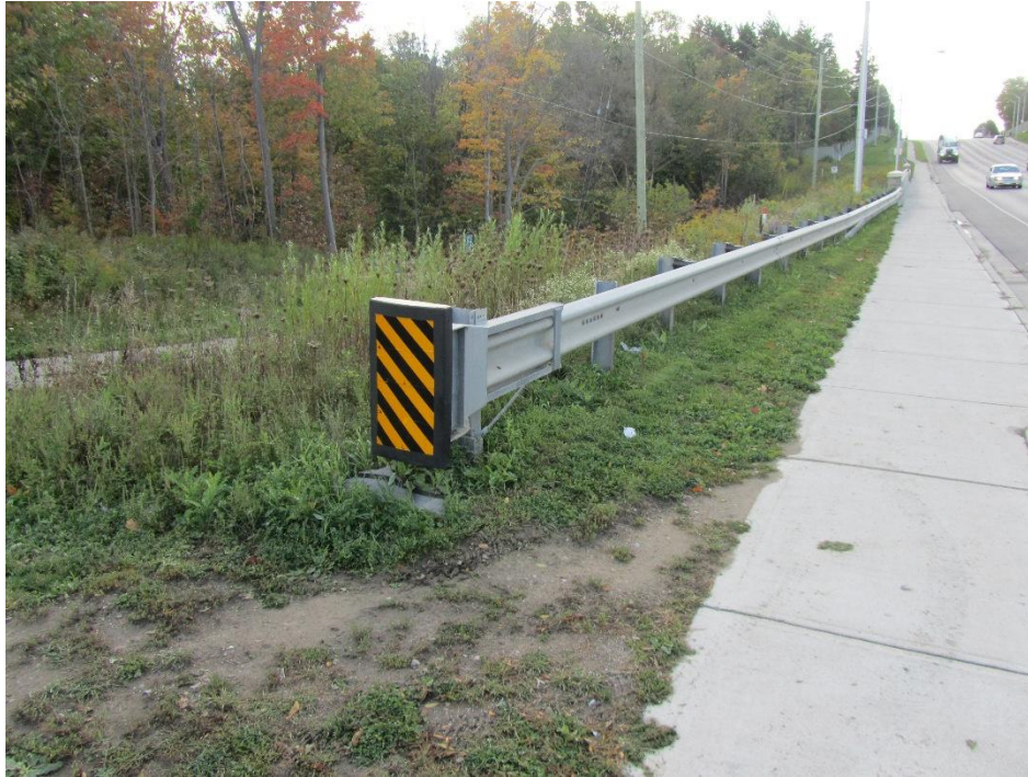
Figure 68: Overall view of north end cap of east guard rail.
