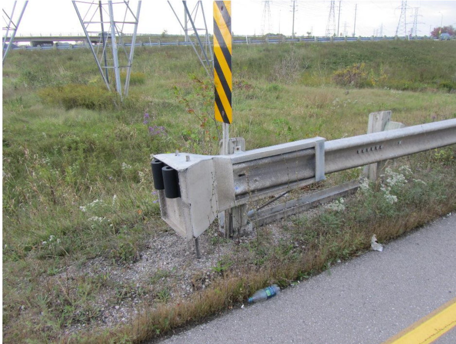
Figure 6: This is likely the original end cap. It is more square.
