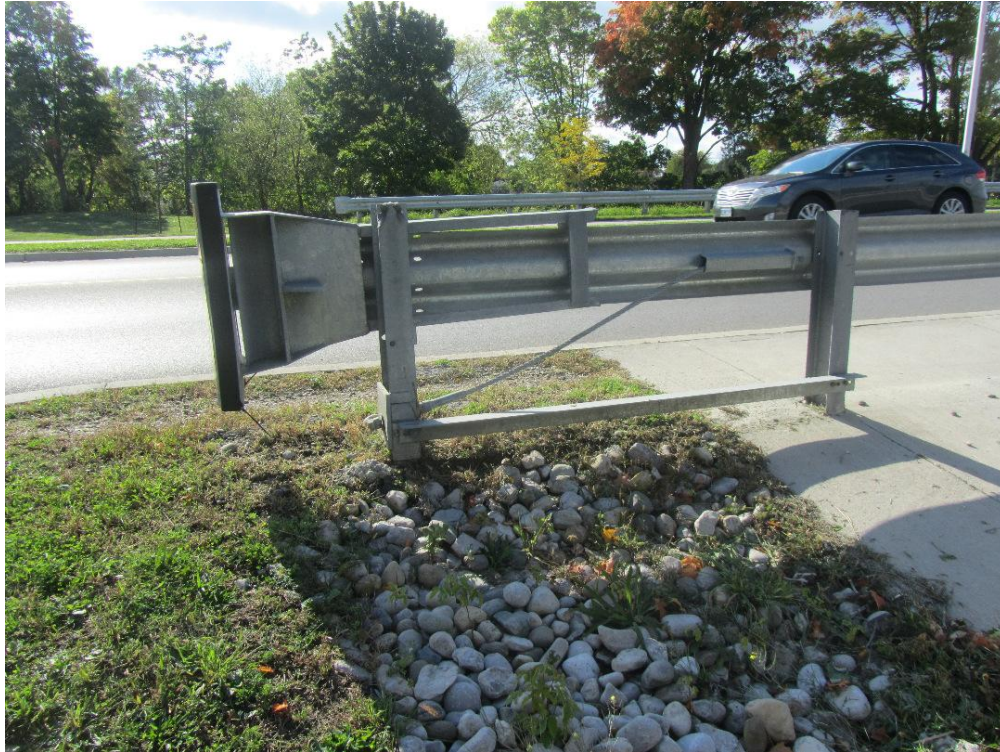
Figure 33: Ditch side view of end cap and channel.
