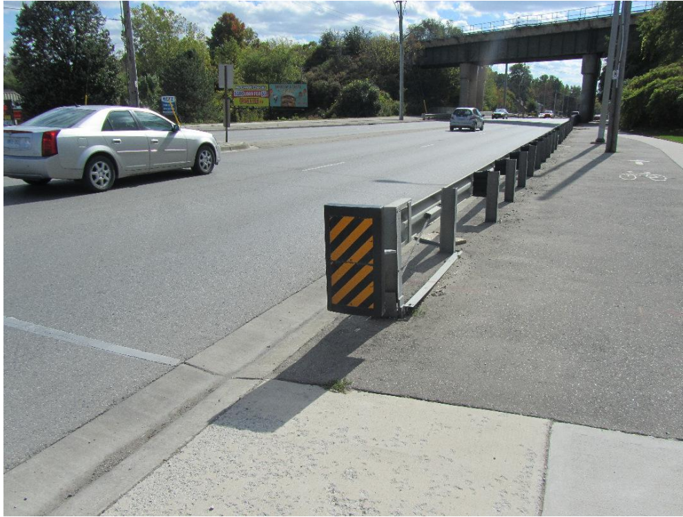
Figure 139: Overall view of 2nd end cap at the west guardrail.
