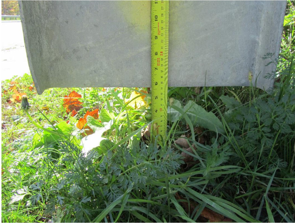
Figure 95: View of base of end plate which is 5.5 inches above the ground.
