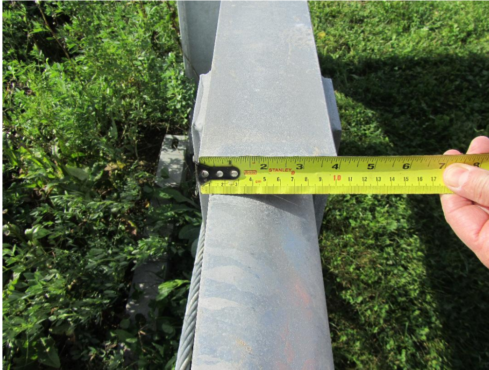
Figure 54: Measurement indicating a 4 inch wide channel.
