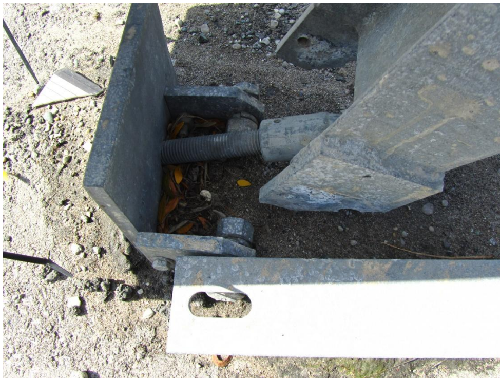
Figure 108: Close-up view showing how the base of the vertical post of the guardrail has been broken free from the bottom anchorage and has been displaced likely as a result of a previous impact.
