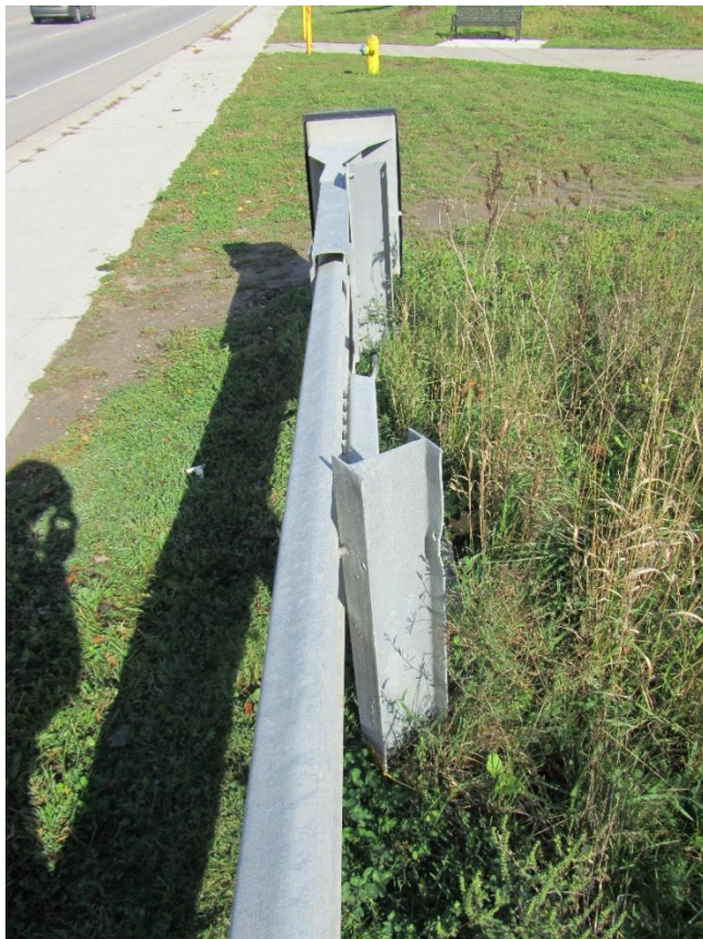
Figure 79: View of peculiar position of anchorage post.
