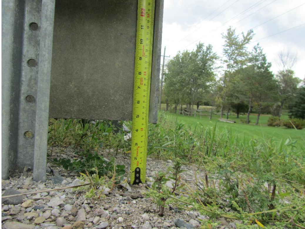
Figure 29: The base of the end plate is just slightly less than 5 inches above the ground.
