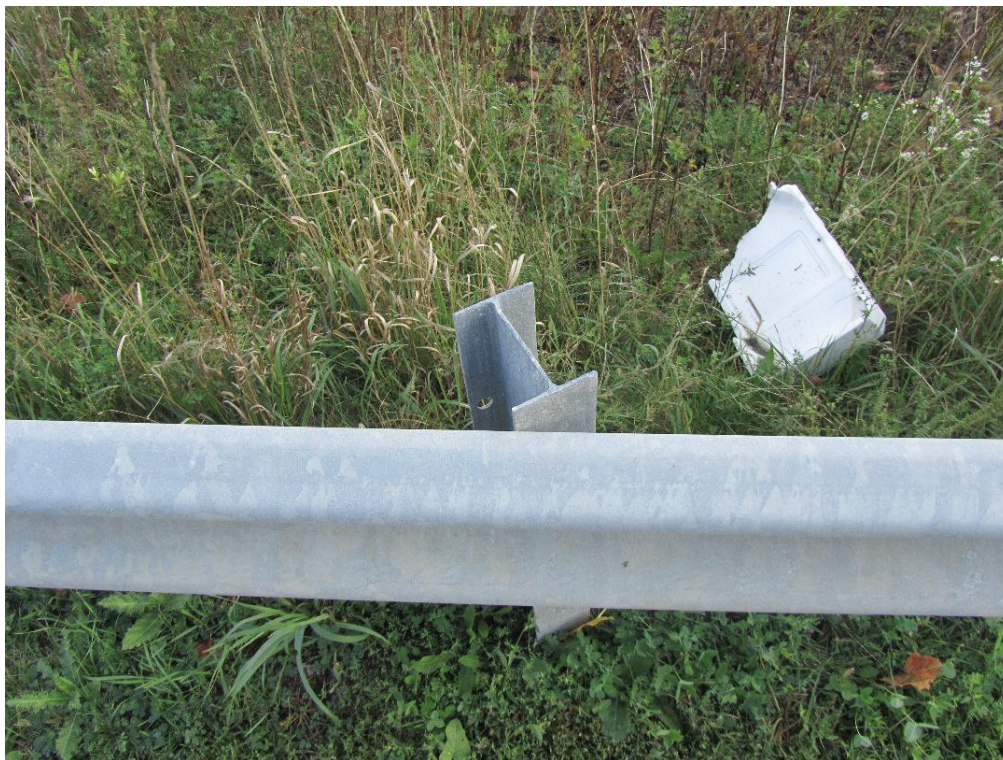
Figure 77: View of peculiar position of the rail anchorage post near the end cap.
