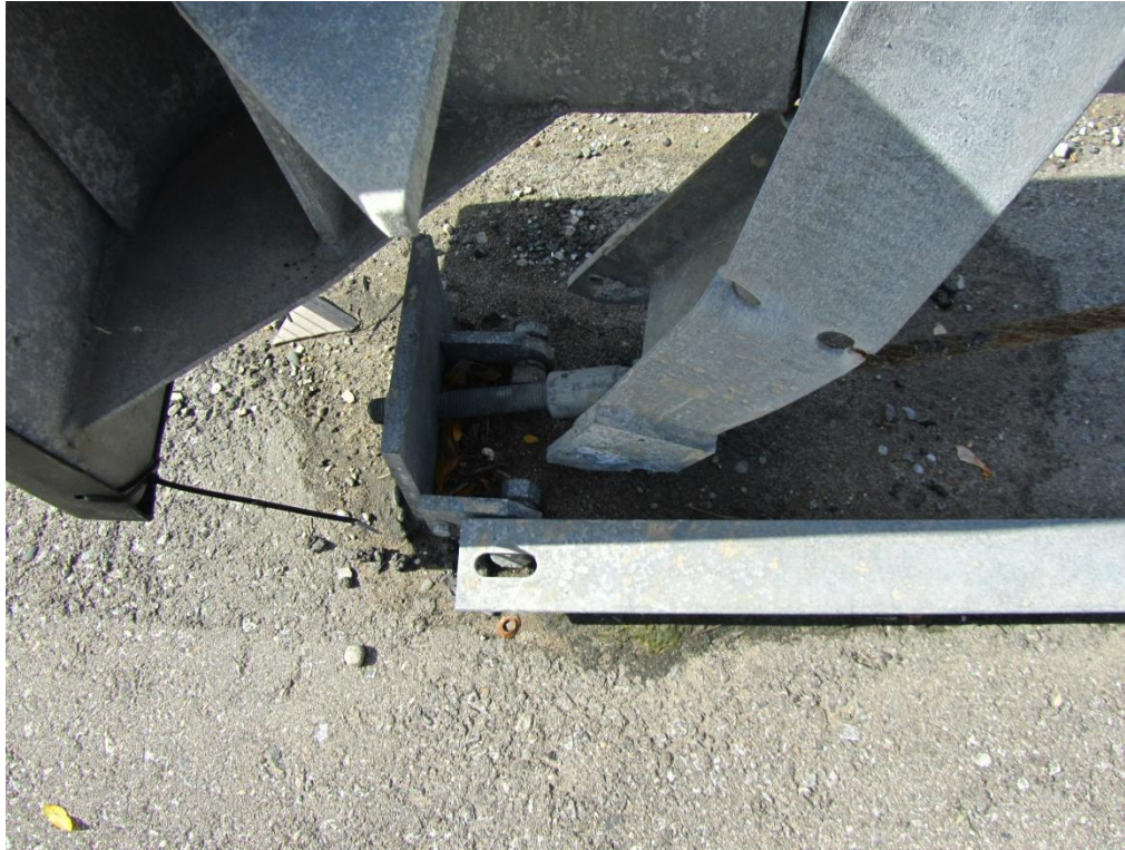
Figure 107: View of the anchorage of the guardrail just behind the end plate showing that the vertical post is deformed and it has sheared away from the anchorage bolts at its base.
