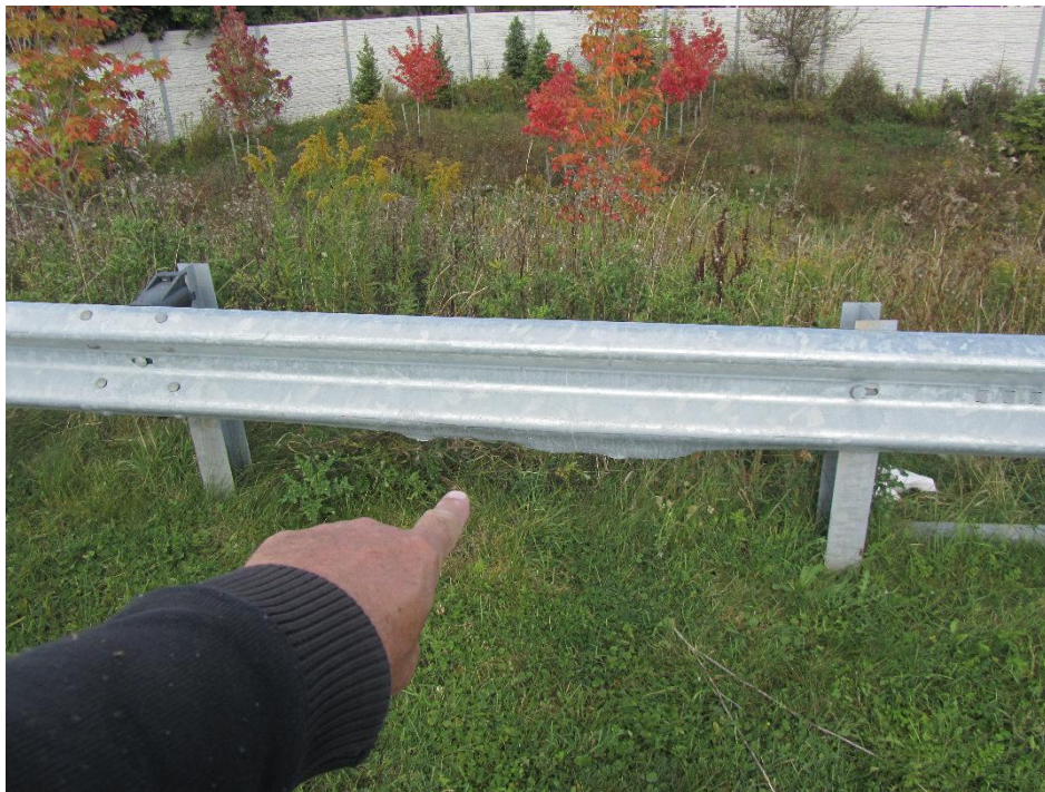
Figure 65: Evidence of damage to the rail near the channel that could affect how the rail passes through that channel.
