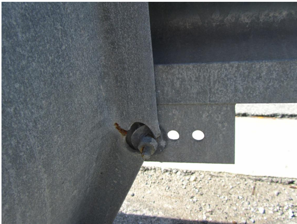
Figure 110: Further evidence of separations between the anchorage post and the guardrail.
