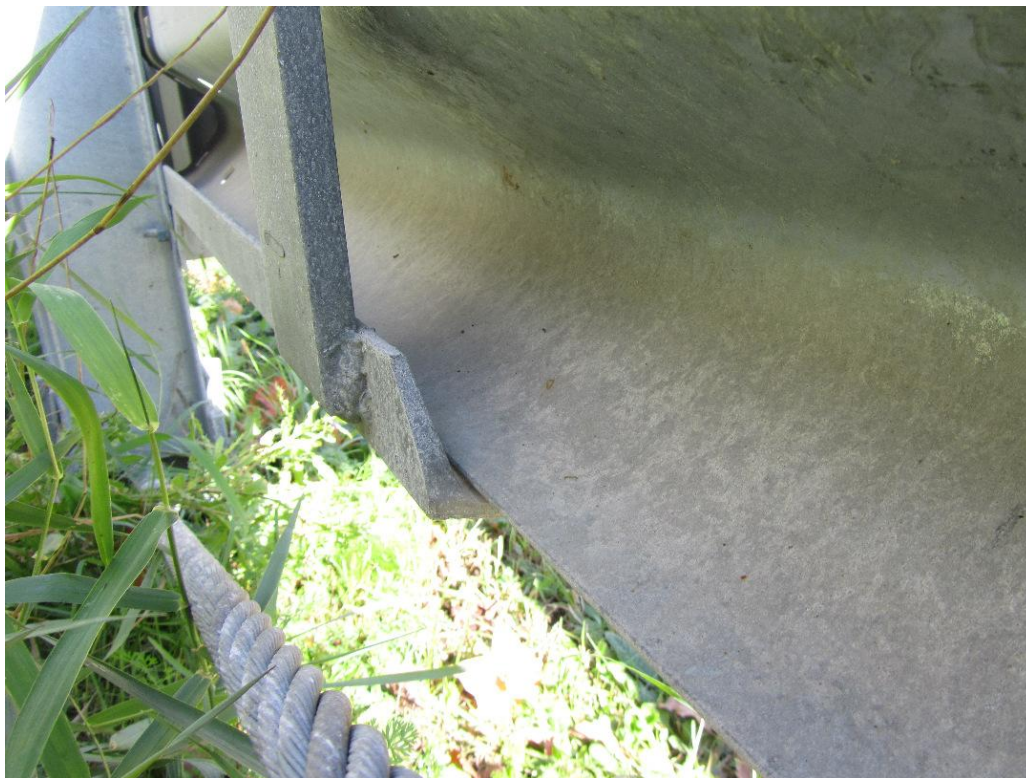
Figure 100: View showing the bottom edge of the rail resting on the bottom of the channel.
