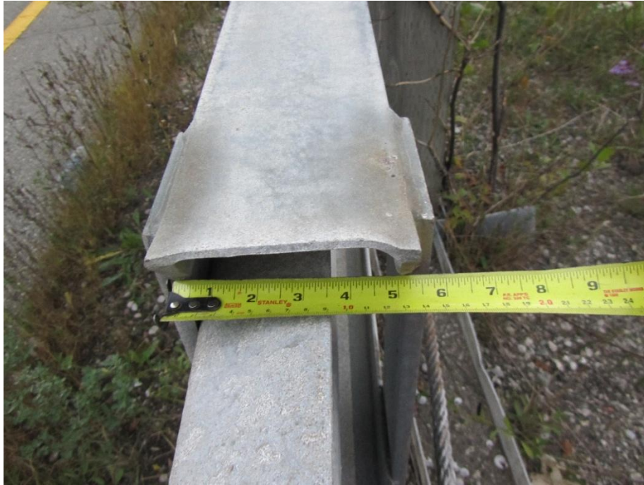
Figure 8: Measurement of channel indicating that it is 5 inches wide.
