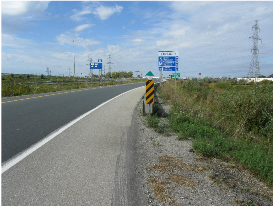
Figure 38: Overall view of hazard marker in front of guardrail end cap.
