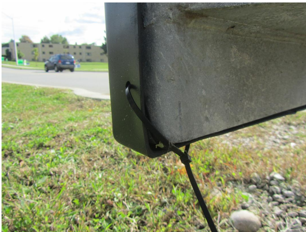
Figure 37: View of plastic tie used to secure the black plastic cover to the end plate.
