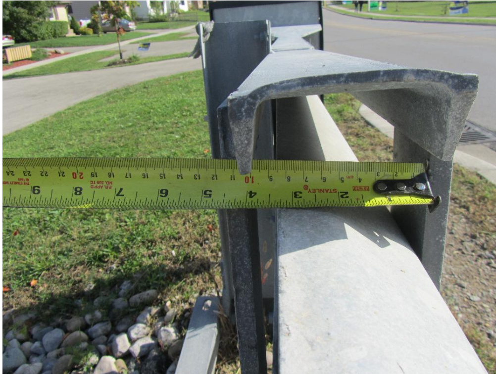
Figure 36: The channel is 4 inches wide.
