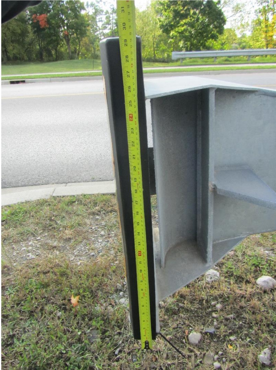
Figure 35: The black cover is slightly taller than 28 inches.
