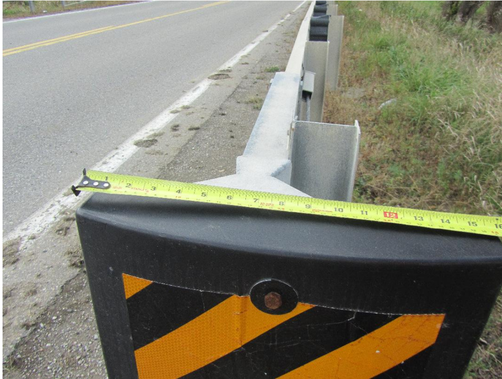
Figure 19: With the black cover attached the end plate is about 16 inches wide.
