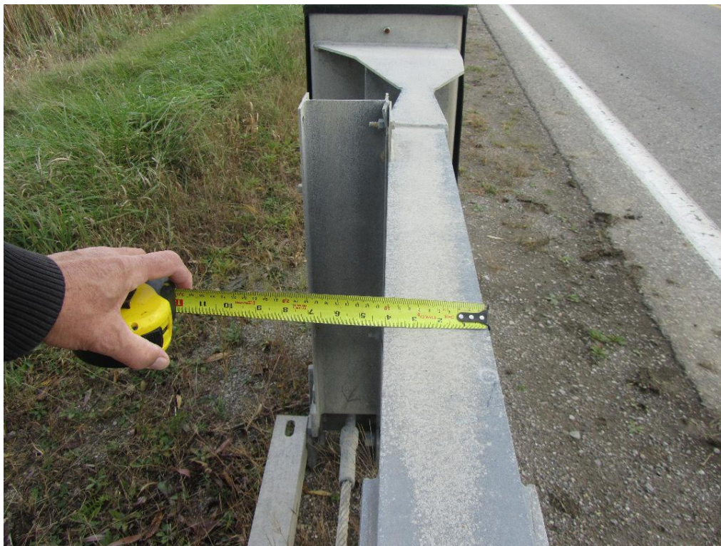
Figure 18: Measurement indicates the width of the channel is 4 inches.
