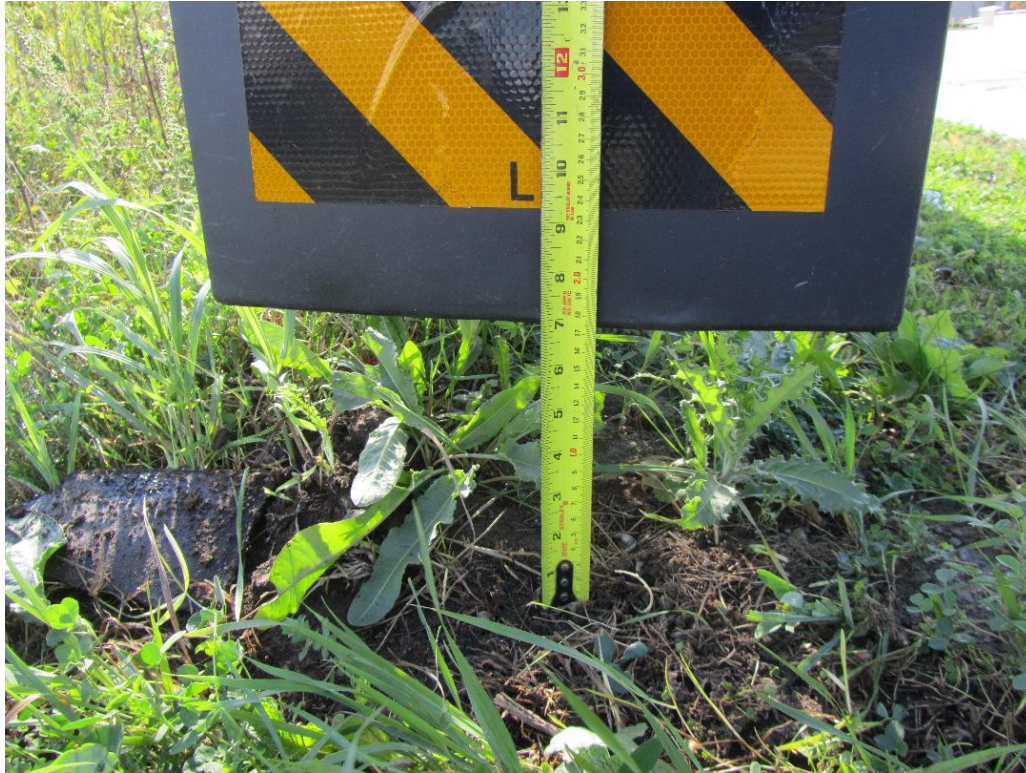
Figure 72: Measurement indicating that the base of the end plate cover is about 7 inches above the ground.
