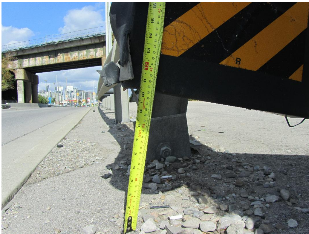
Figure 120: Measurement shows that the street side corner of the cover is about 10.5 inches above the ground.
