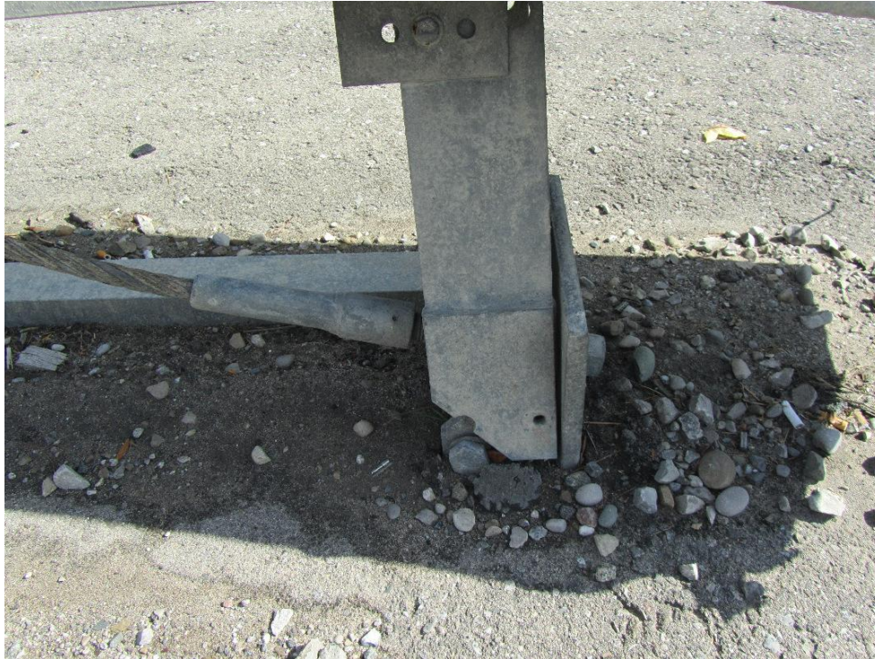
Figure 123: View of anchor post behind the end plate showing that there is a separation between the it and the bottom anchor bolt.
