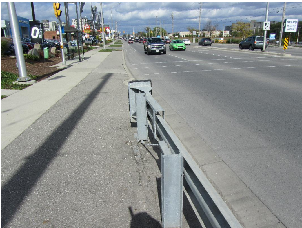
Figure 138: Overall view of the position of the north end of guardrail with respect to the road.
