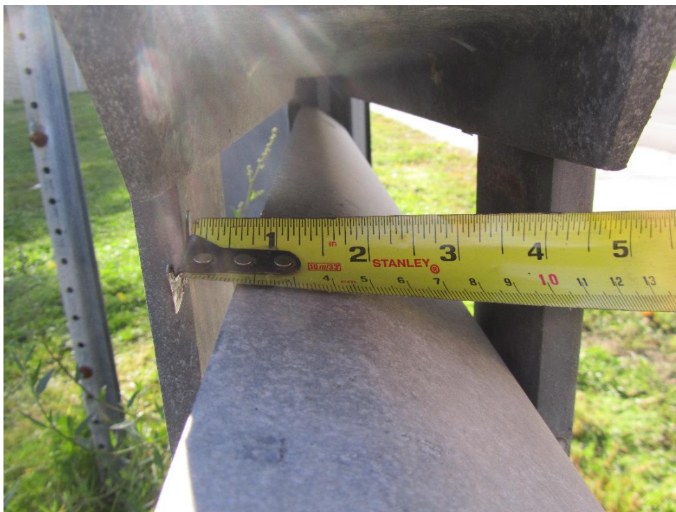
Figure 87: Measurement indicating typical 4 inch wide channel.
