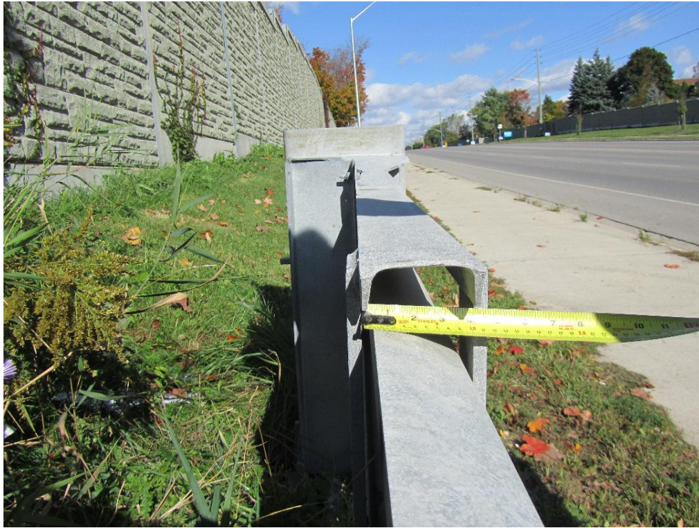
Figure 99: View of measurement indicating that the channel is 4 inches wide and that the rail is positioned at a low level within the channel.
