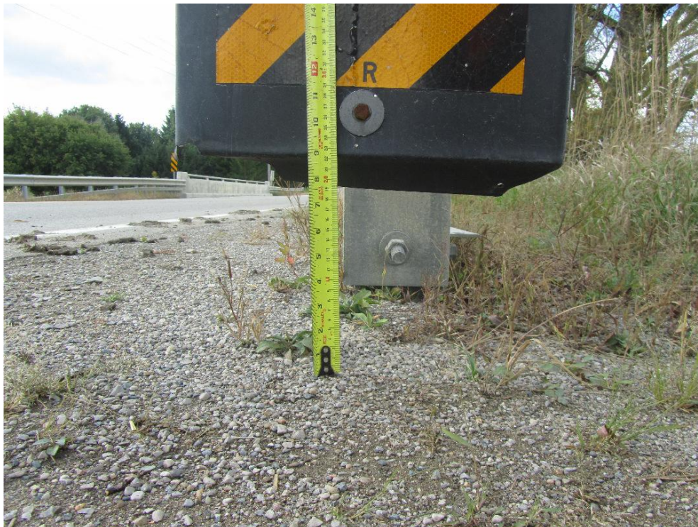
Figure 20: With the front cover attached the bottom of the end plate is about 9 inches above the ground.
