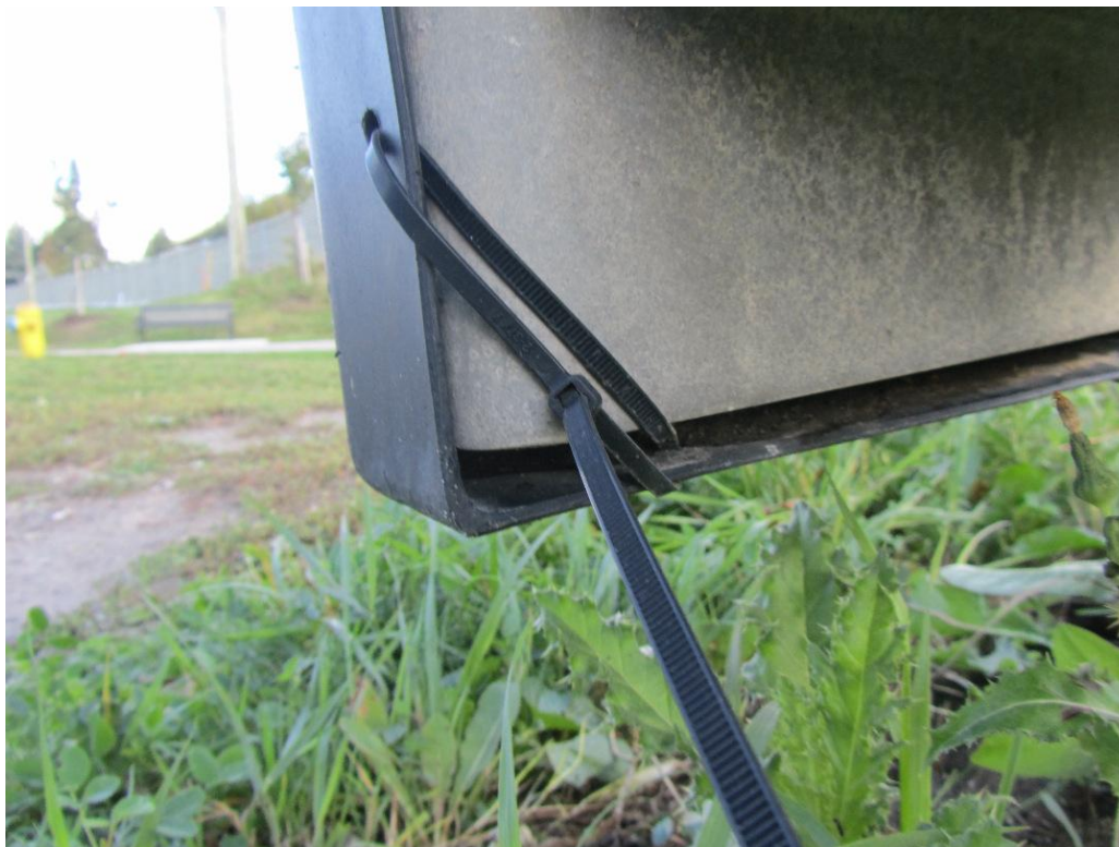
Figure 73: View of typical plastic tie used to secure the cover to the end plate.
