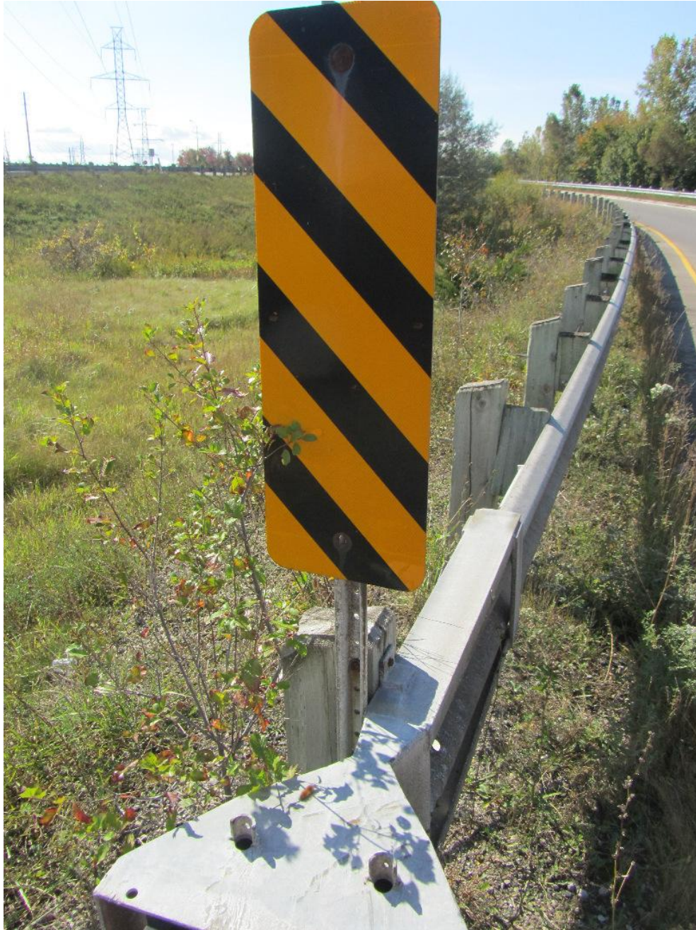
Figure 151: View of post and hazard marker placed in the zone where the end cap's proper collapse along the guardrail must be isolated from any extraneous devices.
