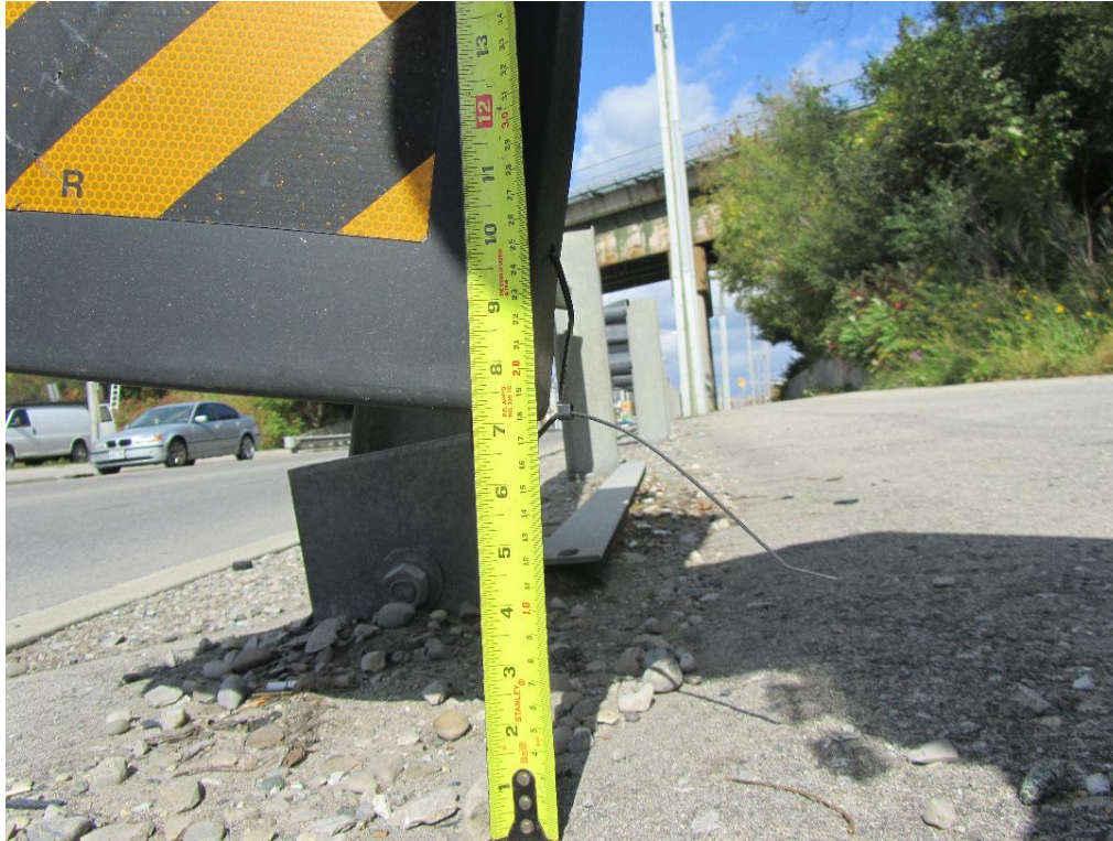
Figure 121: Measurement showing that the ditch side corner of the cover is about 7.25 inches above the ground. This indicates the substantial resting angle of the end plate.
