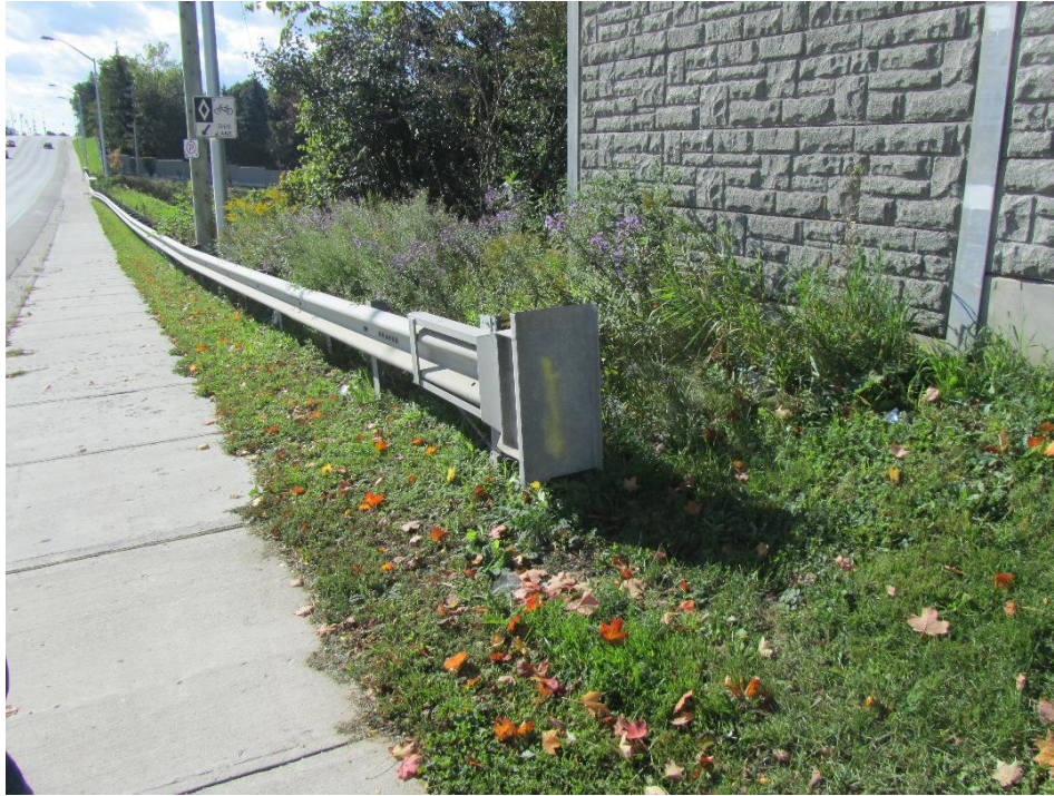
Figure 91: Overall view of north end cap of west guardrail.
