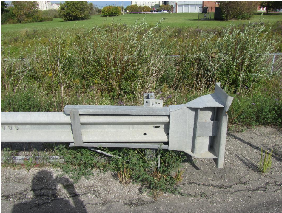
Figure 39: Street side view of end cap and channel.
