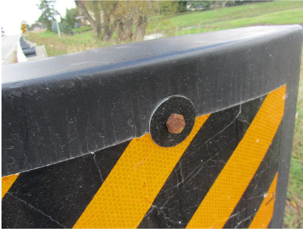
Figure 23: A bolt is used to fasten the black cover to the end plate.
