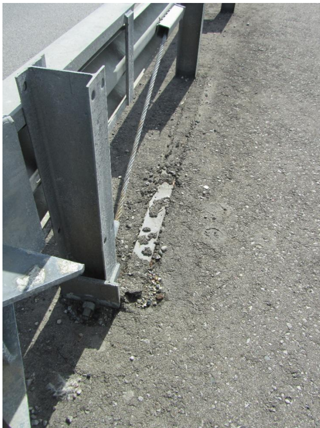
Figure 132: View showing that some asphalt paving has covered the bottom anchorage plate.
