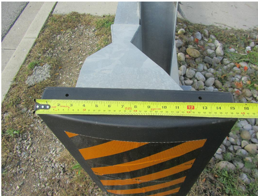
Figure 34: The black cover of the end plate is just over 15 inches wide.
