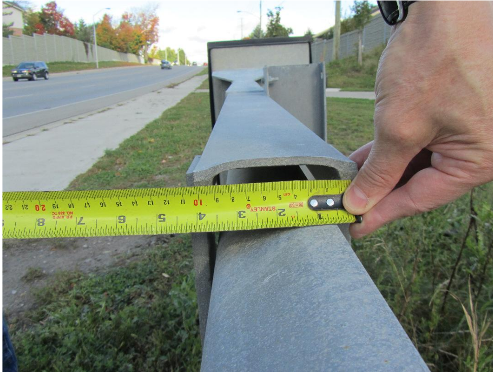
Figure 74: Measurement showing that the channel is the typical 4 inch width.
