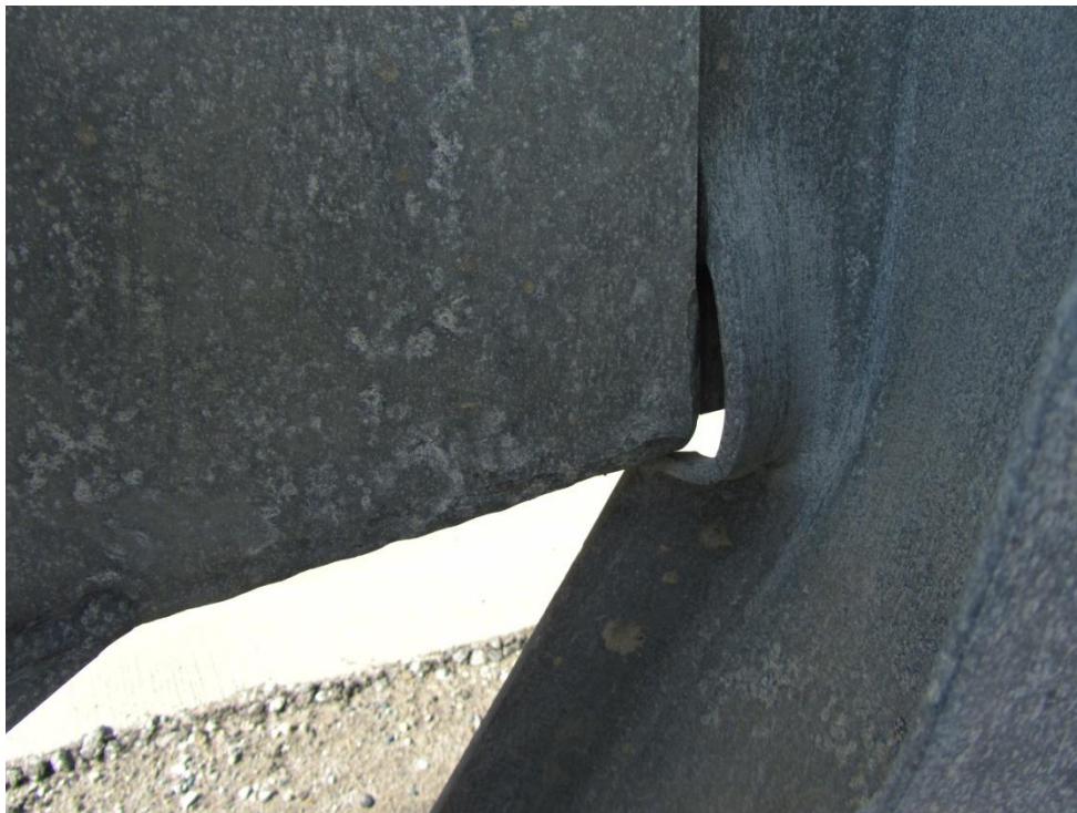
Figure 112: Close-up view of damage to the vertical post from contact with the back of the end plate which has been displaced, likely by an impact.
