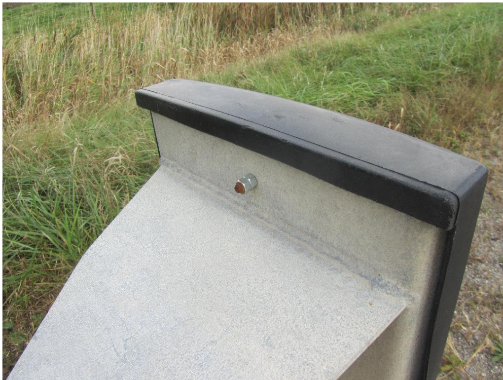
Figure 22: Efforts to secure the black cover to the end plate are evident here as a bolt holds the cover to the plate.
