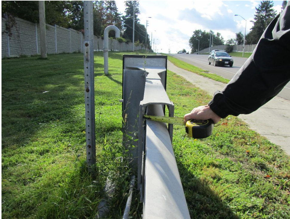
Figure 86: View showing measurement being taken of the width of the channel. Note that the rail is positioned low within the channel.
