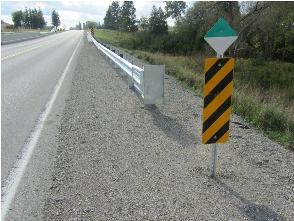
Figure 149: View of post and hazard marker placed in front of the guardrail end plate.
