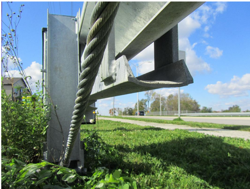
Figure 55: View showing the rail positioned high within the channel.
