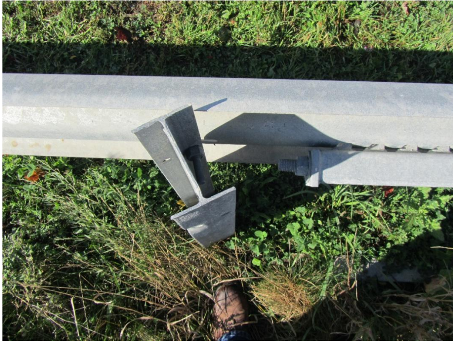
Figure 78: View of peculiar position of the rail anchorage post near the end cap.
