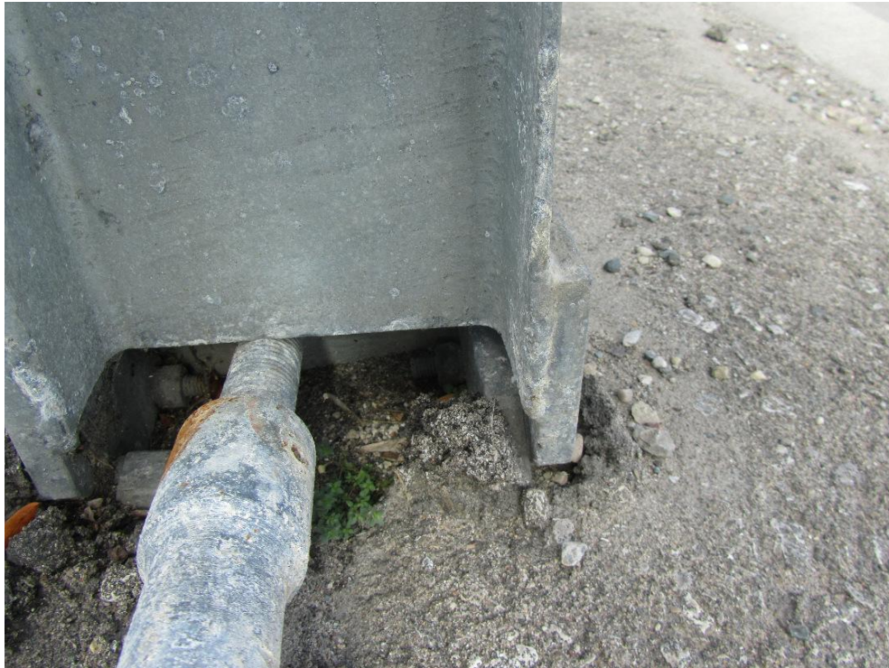
Figure 133: Closer view at the base of the vertical anchor post near the end plate where the higher asphalt pavement might interfere with the separation of the post from its "tight fit" design.
