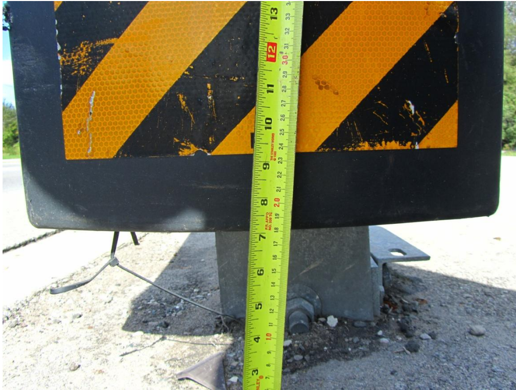
Figure 105: Measurement indicating that the base of the cover is 7 inches above the ground.
