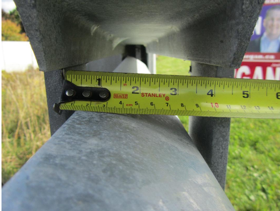
Figure 64: Measurement indicating the width of the channel is 4 inches.
