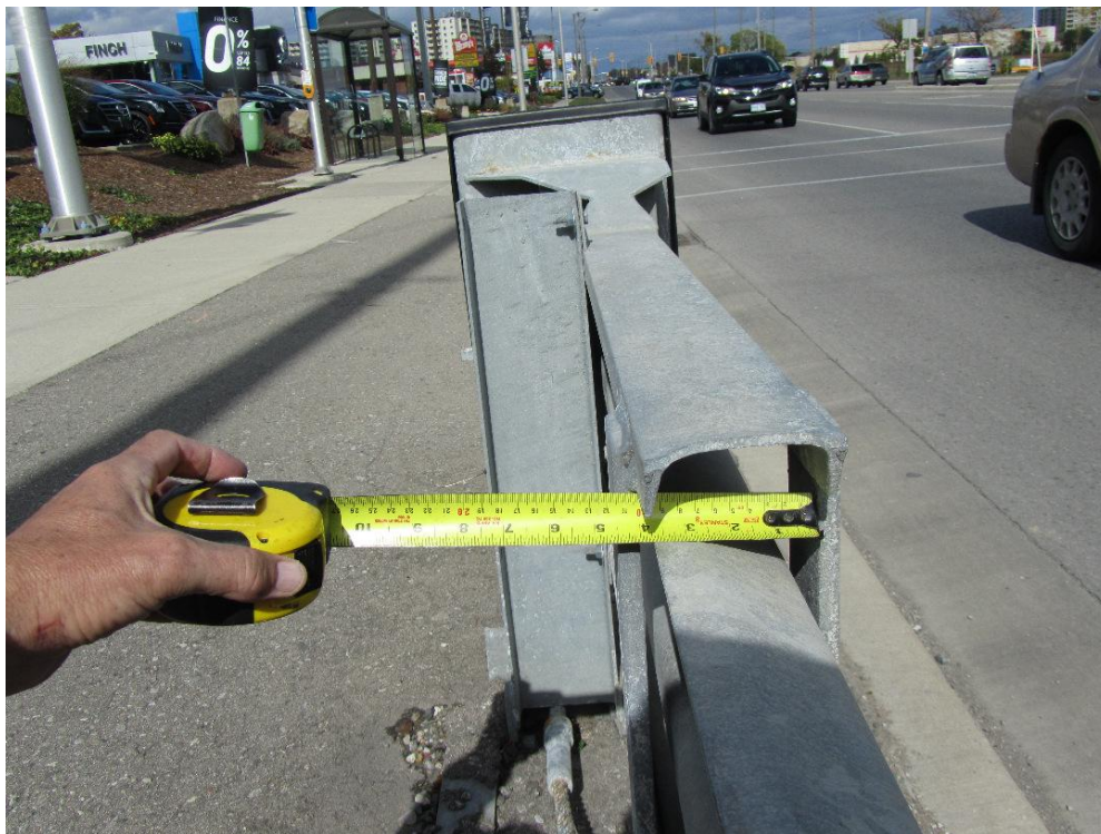
Figure 134: View of measurement indicating that the channel is 4 inches wide. Note that the rail is sitting low within the channel.
