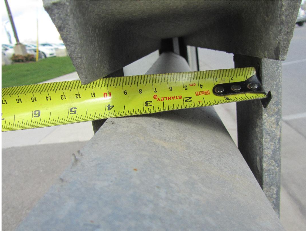
Figure 145: Measurement indicating that the channel is 4 inches wide.
