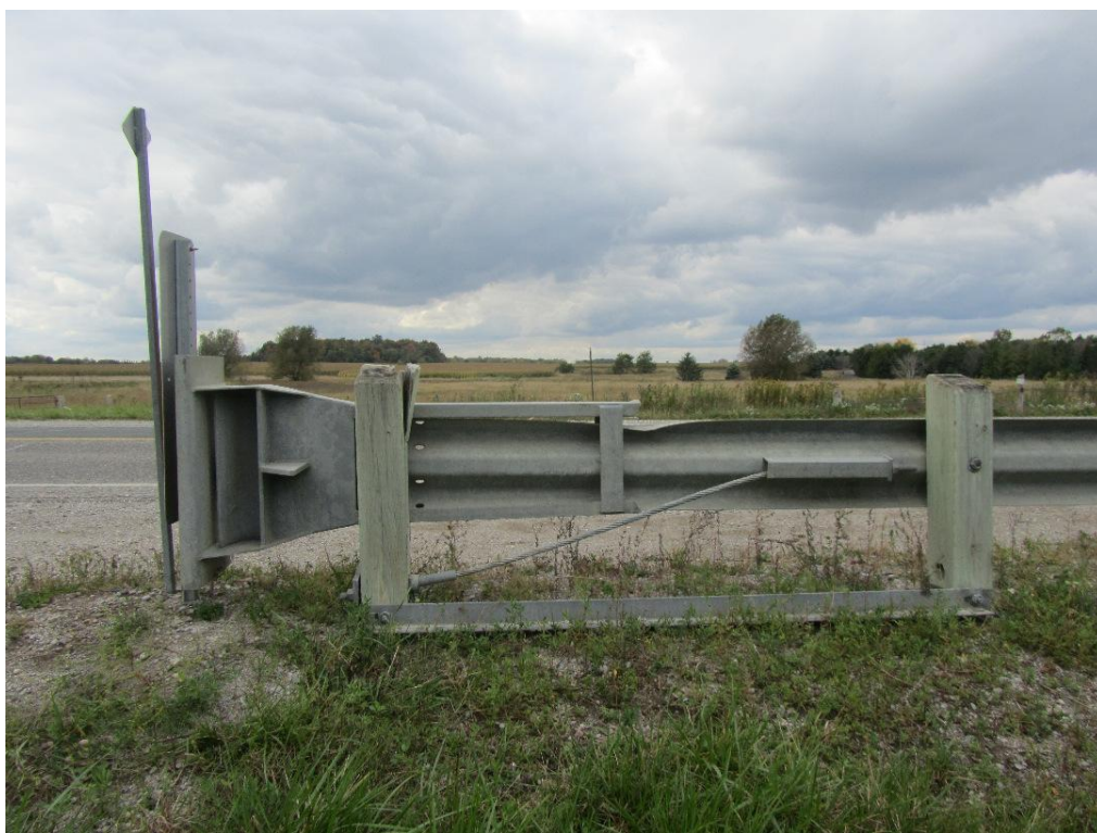
Figure 26: Ditch side view of end cap and channel.
