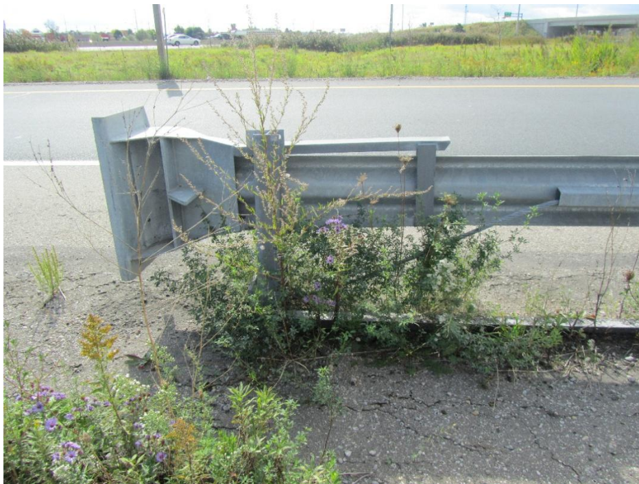
Figure 40: Ditch side view of end cap and channel.
