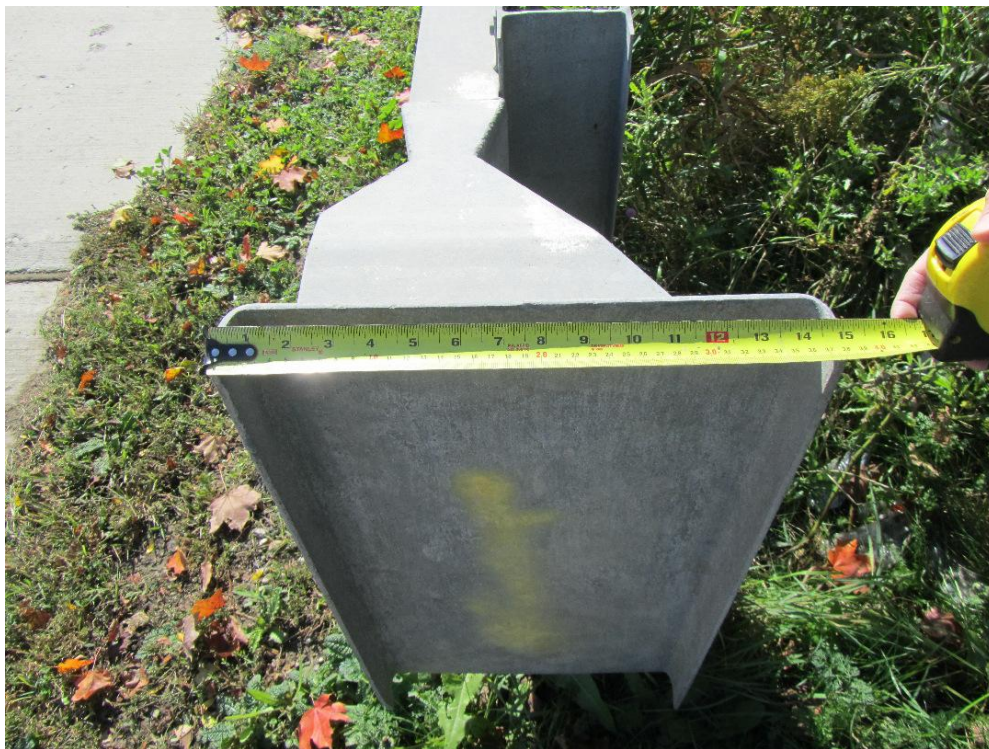
Figure 94: Measurement of north end plate (15 inches wide) which is missing its cover.
