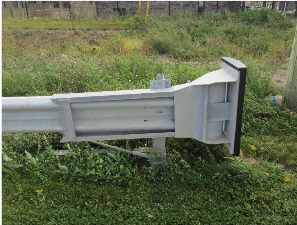
Figure 46: Street view of channel and end plate.
