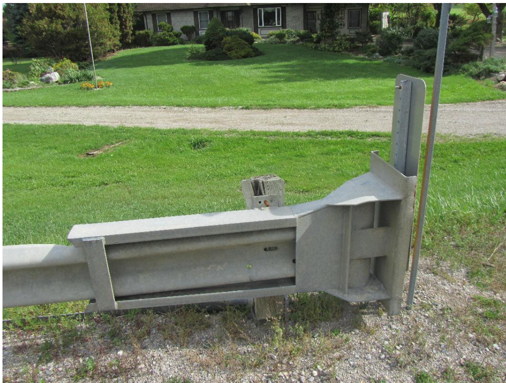
Figure 25: Street side view of the end cap and channel.
