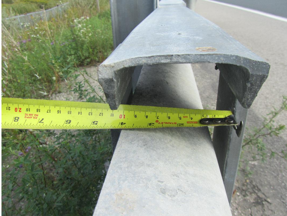
Figure 44: Measurement indicating the channel is 4 inches wide.
