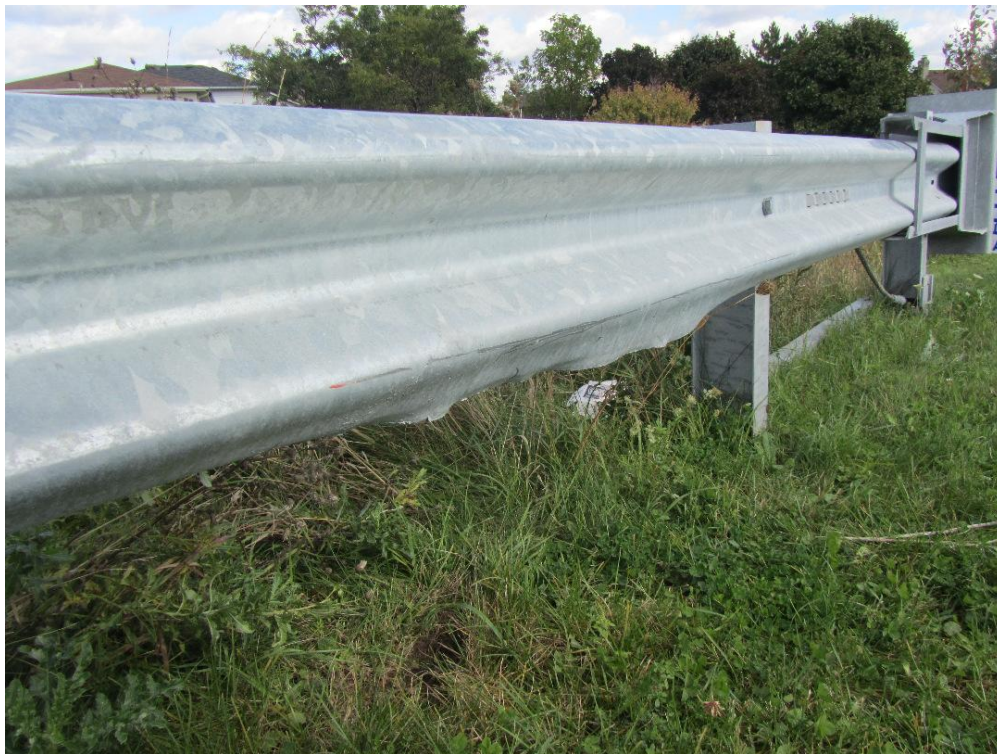
Figure 67: Photo indicating that scrapes also exist to the front face of the rail in the area of the deformation.
