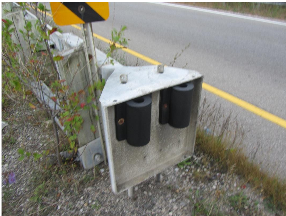
Figure 7: The end cap appears to be missing its front cover.
