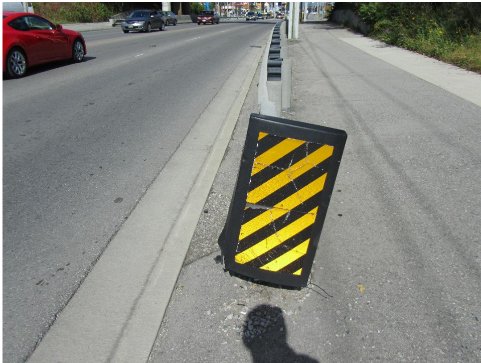
Figure 116: Closer view showing that the end plate hidden by its cover, is at a non-vertical angle.
